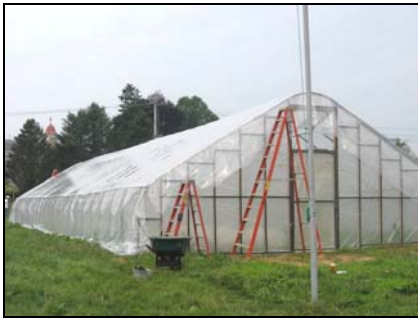
Completely “skinned” tunnel (photos by Mira)
